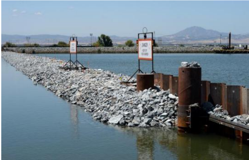
A levee road on Bradford Island, Calif. (Susan Tripp Pollard/Bay Area News Group)
